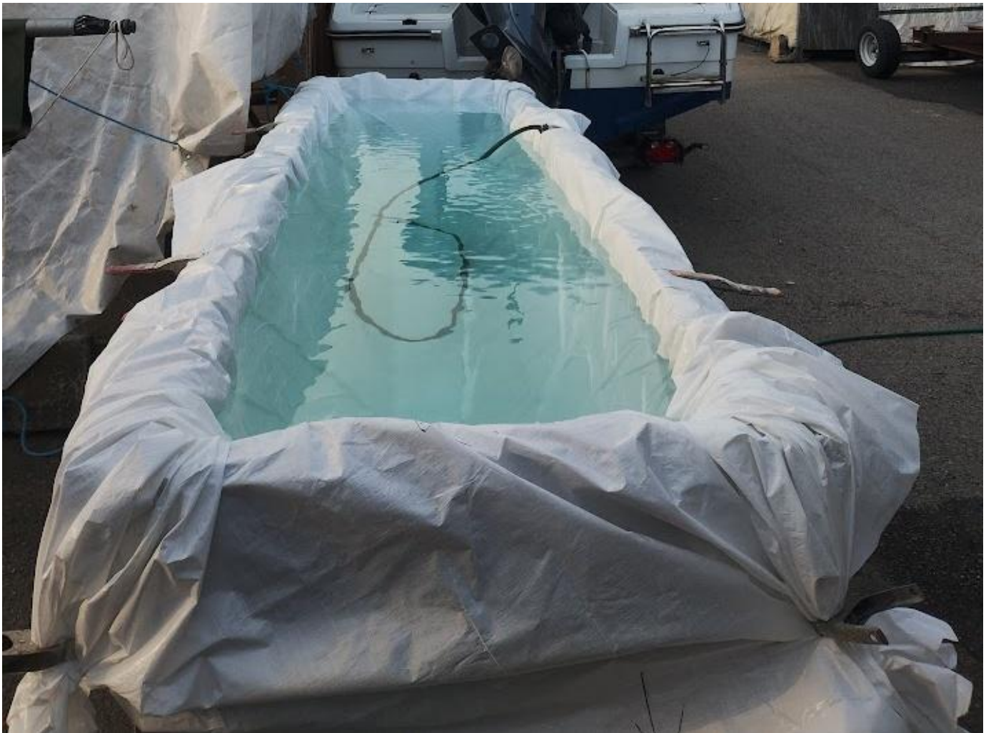
Step 5 fit the plastic liner and fill with water
